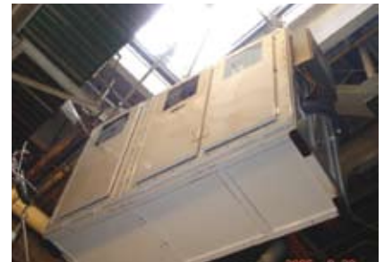
A GOSFERN™ control system is lowered into the engine room.
