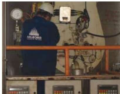
Service and upgrading of burners and safety/control systems
