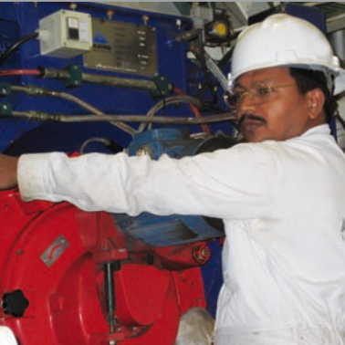
Aalborg Industries' own design of rotary cup burners (KB™) or the steam atomizing types (KBSA™) can be used on the MISSION™ OM-TCi boiler. The burners have a long life cycle and are easy to maintain.
